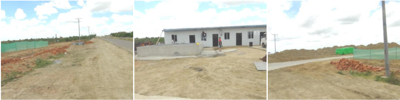
(The construction progress recorded on 1.5.21)
